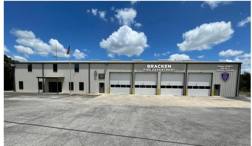
Provided this 1999 constructed steel framed building with a needed electrical and h-vac upgrade to meet current code, while also rearranging much of its space to better accommodate operations and crew living areas.
