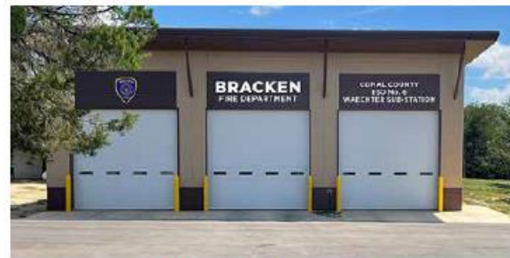
Waechter Substation, Corner of Hwy 1863 and Delafield Drive, New Braunfels, TX 78132 Added equipment-apparatus-bays, permitting 24/7 operations and is helping to improve service response
